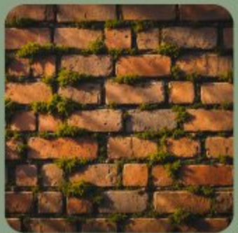
Walls and Brickwork
